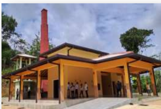
Construction of crematorium building and external work of Neluwa Pradeshiya Sabha Neluwa P.S. Southern Province
