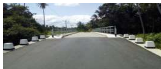
Bridge No. 5127, Kurunagala Kosdanda Canal Bridge
