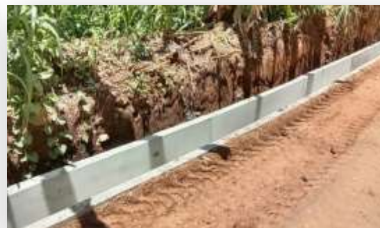
Construction of U type side drains on Welanhinna - Kirigalpotta road in Badalkumbura PS area of Monaragala District
