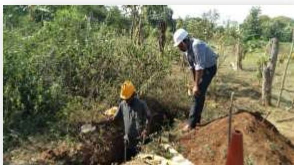
Pipe laying works at Puthiavellar Sinnakulam Drinking Water Project, Vavuniya South Tamil Divisional Secretariat, Vavuniya District
