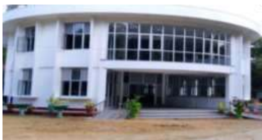
New OPD – Damana Divisional Hospital
