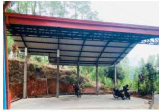
Repairing the Kalawana Pradeshiya Sabha Office building and the vehicle park Kalawana P.S. – Sabaragamuwa Province
