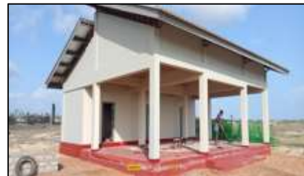
Construction of Tourist service centre with sanitary facilities at Casurina Beach
