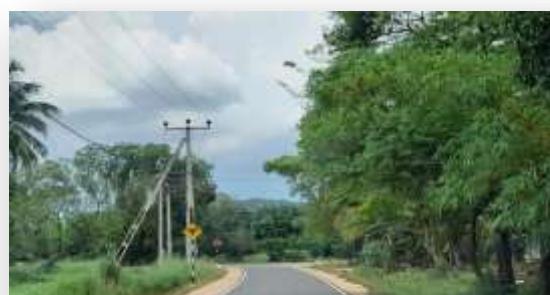
After improvement of Himbutugollewa – Thammannagama – Kolongaswewa Road in Galenbindunuwewa Divisional Secretariat of Anuradhapura District
