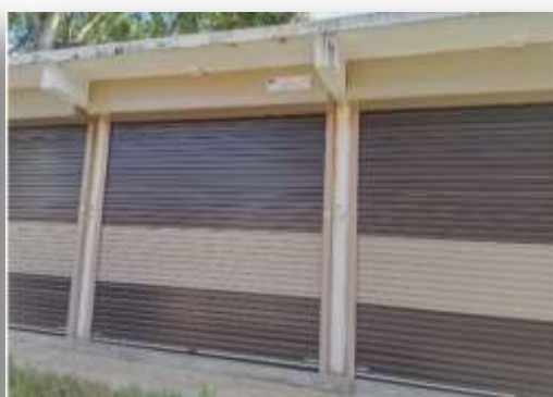
Construction of stalls for the Karametiya weekly fair Meegahakiwula P.S. Uva Province
