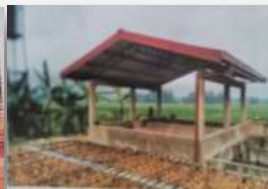
Construction of Gully Waster Treatment Center in the Pannala Pradershova Sabha
