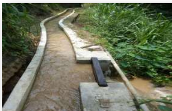
Rehabilitation of Mahantewela Anicut and Canal in Kandekatiya PS Area of Badulla District
