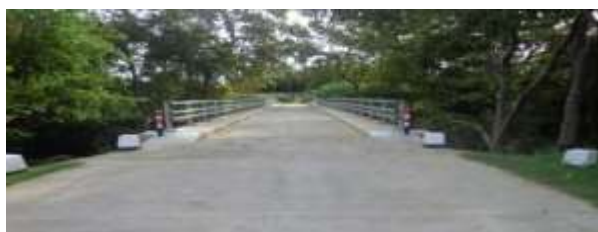
Bridge No. 5115, Thellulla Bridge over Monaragala Kirindi Ova
